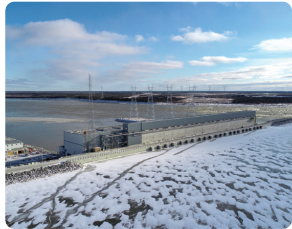
Keeyask generating station
