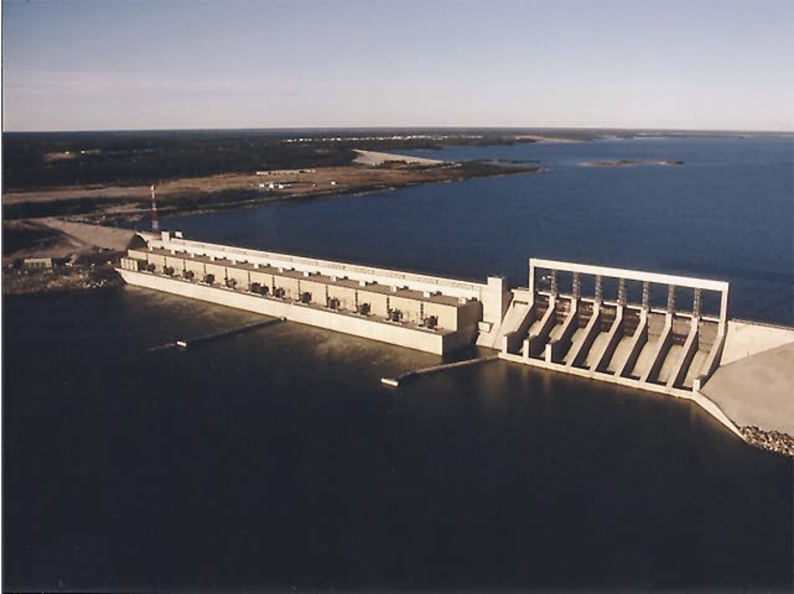
Photograph 1: Kettle Generating Station
